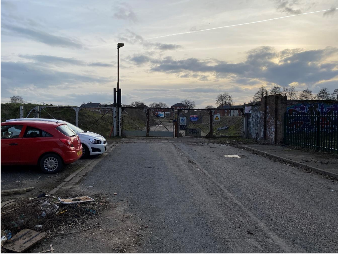
Access into the site
