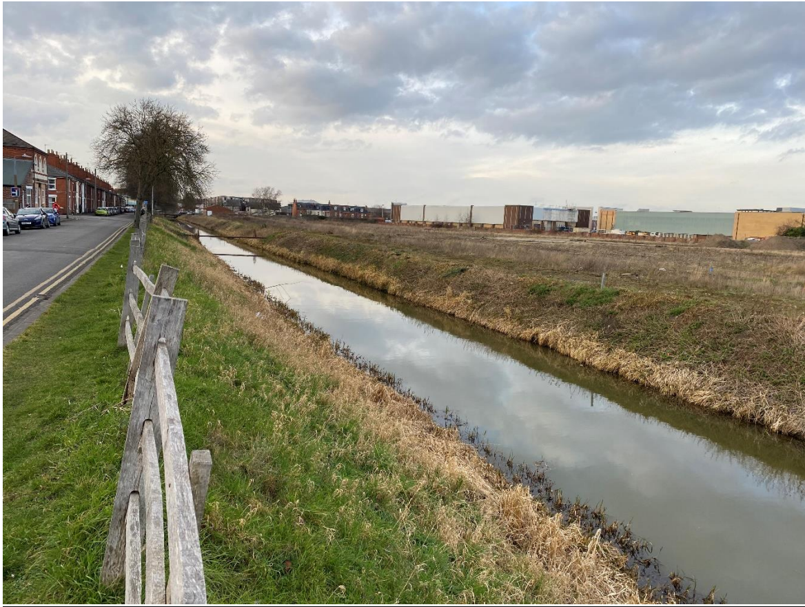
Boultham Pump Drain
